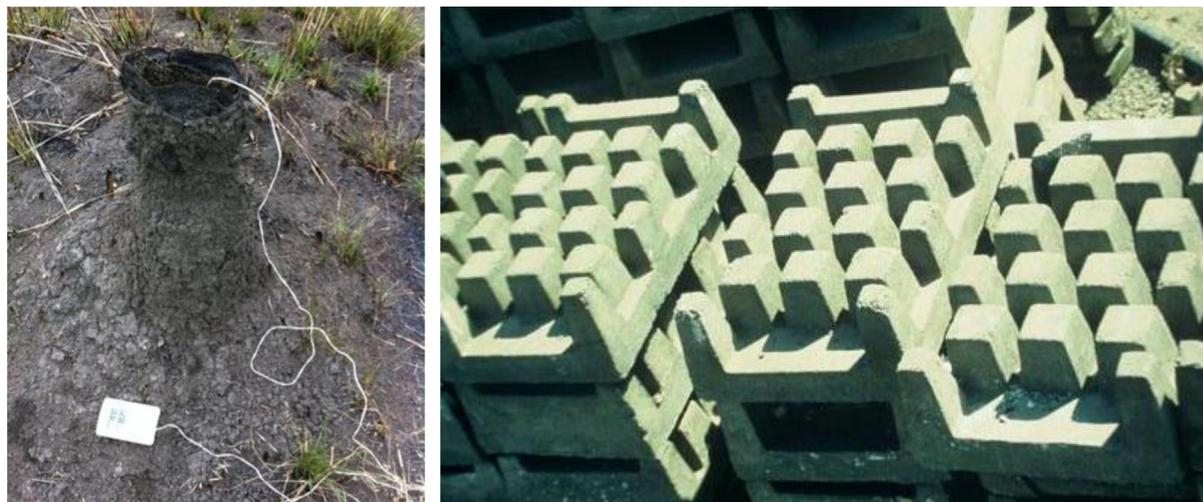
**Fig. 4.** Temperature measurements of termite mounds carried out by Mick Pearce (left), CC-SA-BY Licence, Mick Pearce. (b) Heat exchange floor under construction, abstraction of the biological principles of termite mounds, CC-SA-BY Licence, Mick Pearce.
